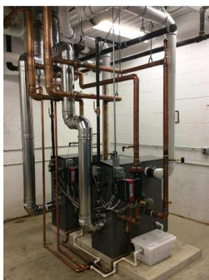
Two new boilers have been installed. Insulating the pipes will be completed soon. All are invited to visit the boiler room located on the lower SGD wing to the left of the elevator. Just ask for a key from the front office. Questions? Contact Interim Administrator Ed Lynn at [ed@uuaa.org](mailto:ed@uuaa.org).
